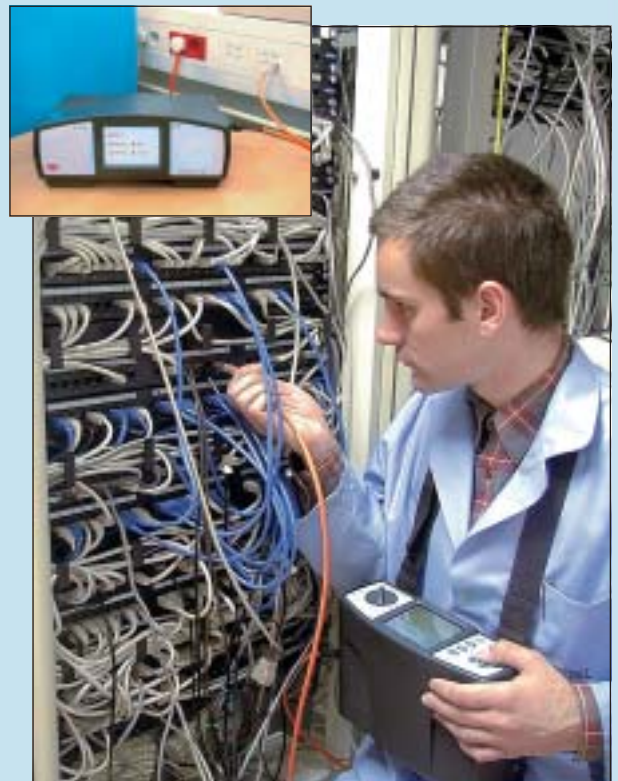
Certification of Cat 6 installations. Performance tests of all installations up to 350 MHz.
